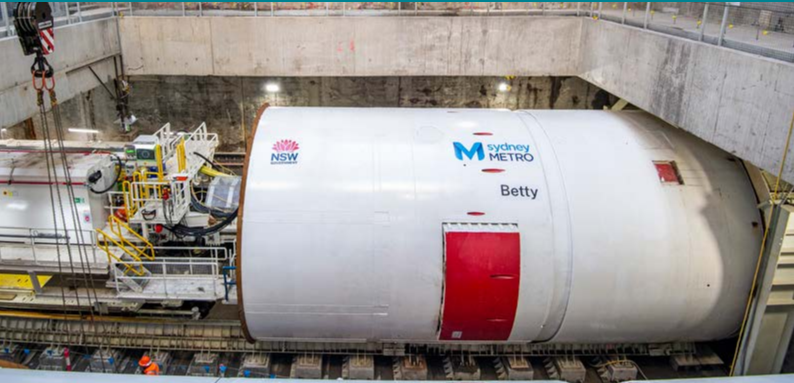
Tunnel boring machine (TBM) Betty in the Rosehill launch box.
