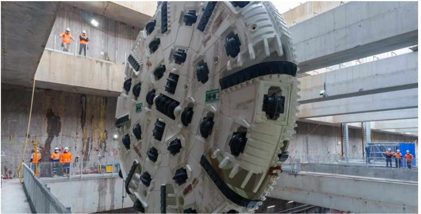
Tunnel boring machine (TBM) Betty cutterhead lowering.
