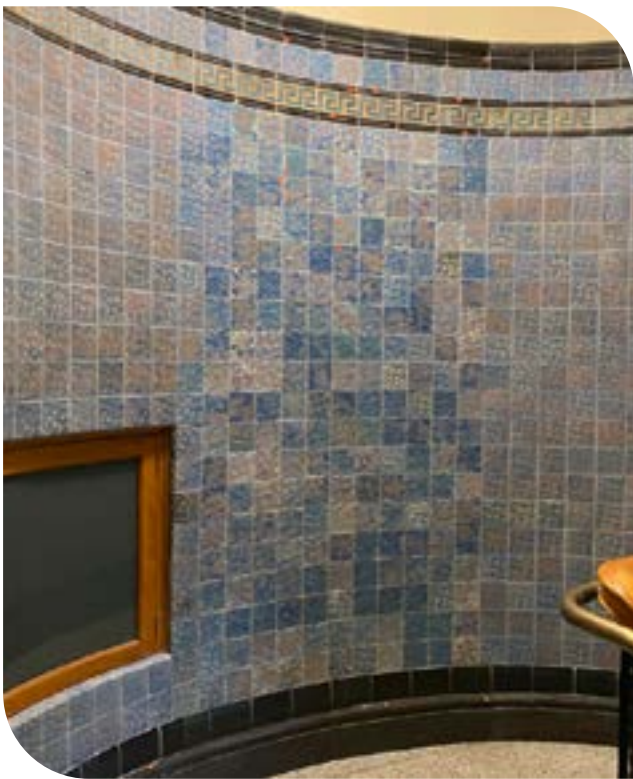
Infilled wall with salvaged and new.
